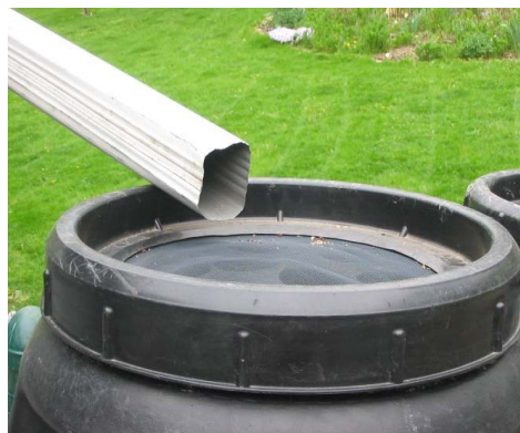
Downspout elbow used to direct water into the barrel. Can also use optional "Flex Elbow" to direct the water from the downspout.
