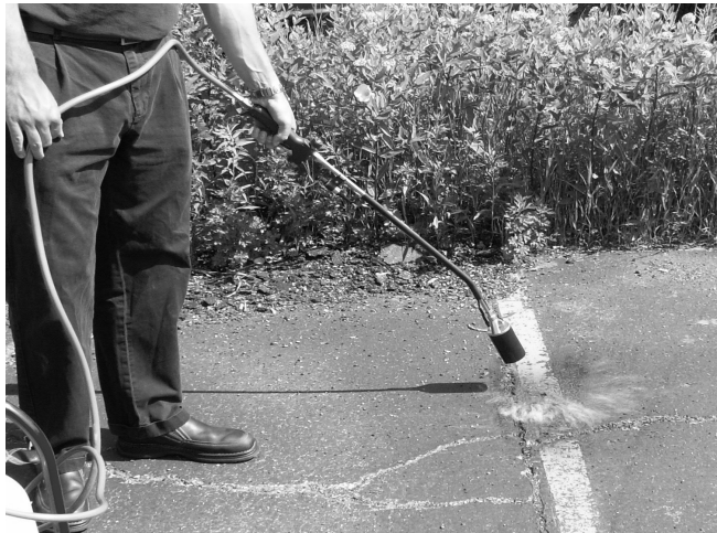
Removing Paint
