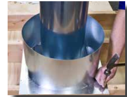
6. Slip insulation shield over chimney until base sits squarely on framed opening or nests in the support box. Nail to opening or screw to box.
