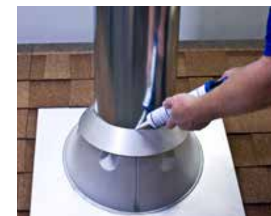
13. Apply high temperature silicone sealant where storm collar will meet chimney. Slip storm collar around chimney and slide down. Seal with high temperature silicone sealant.
