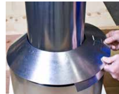
7. Wrap insulation shield collar around chimney. Slide it down to the shield.
