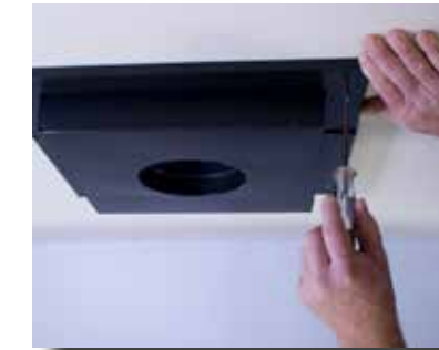
4. Screw the support box trim to the ceiling.
