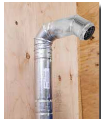
10. Attach horizontal cap to the top elbow.
