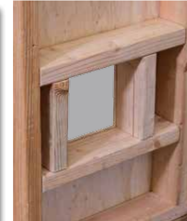
2. Cut and frame wall penetration.
