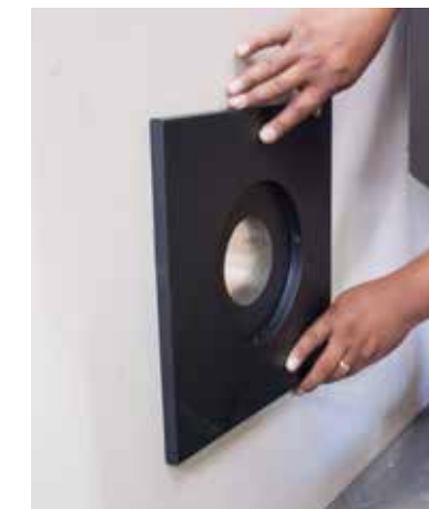
6. Level and attach inside portion of the wall thimble to the wall.
