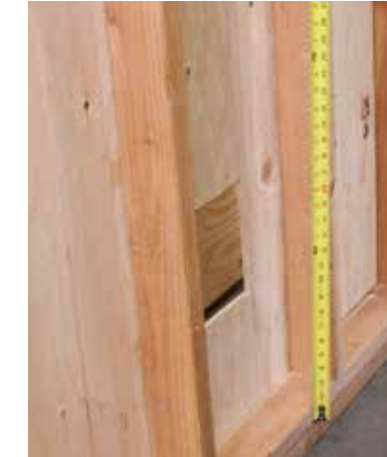
1. Locate appliance and penetration through wall.
