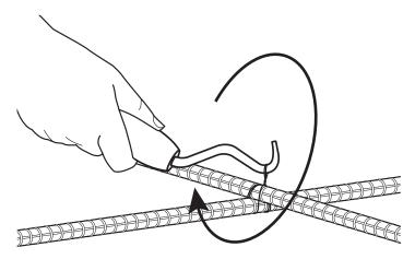
Fold the loop down to keep it from nearing the surface of the concrete.
