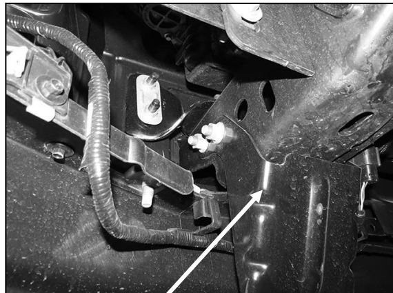
(Fig 6) Driver/left frame extension pictured
