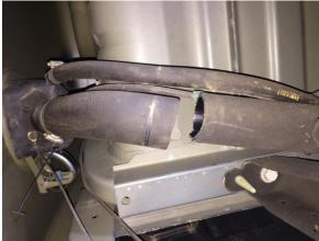
9) Install the adaptor as horizontal as possible with the control valve upright. Secure the adaptor tightly with the hose clamps.
