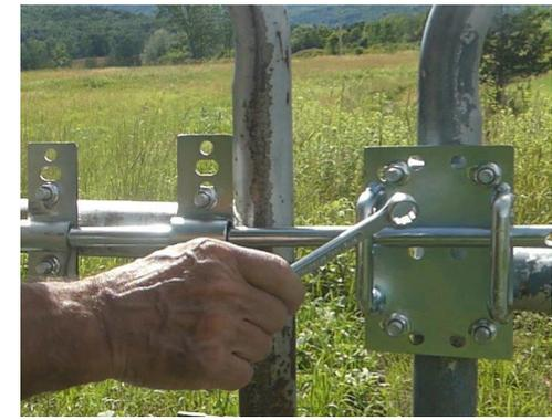
No welding – a wrench, or ratchet, and about 20 minutes gets the job done. Over time, gates and posts tend to sag and tilt. This feature makes it easy to make adjustments as necessary.
