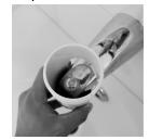
9. Screw the top of the tub spout diverter back onto the bottom piece. Firmly tighten over your tub spout's tee. (The tee is what you pull to divert water to your shower.)
