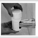
10. Screw the larger end of the hose onto the outtake of the tub spout diverter. (The outtake is on the bottom of the
