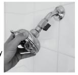
4. Keep the valve lever in the ON position (180° or parallel to pipe) to operate your shower normally. This valve stays installed.
