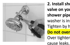
2. Install shut off valve on your shower pipe. Ensure washer is installed. Tighten by hand. Do not over tighten! Over tightening will
