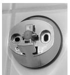
12. Screw smaller (nut) end of hose into shower diverter (ensure circular rubber washer is in place in hose); tighten with pliers
