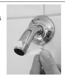
3. Screw shower diverter nut on shower pipe over plumbers tape; tighten with pliers. (Spin diverter clockwise to tighten if loose)
