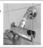
4. Cut two more 2-3 inch pieces of plumbers tape and wrap each piece around remaining two diverter threads
