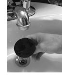
9. Place suction cup on wall (with metal pin running horizontally); firmly press suction cup to wall
