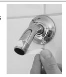
3. Screw shower diverter nut on shower pipe over plumbers tape; tighten with pliers. (Spin diverter clockwise to tighten if loose)
