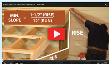
Typical Canopy Framing Detail
