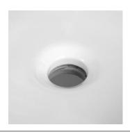
6. Wipe off the excess silicone around the drain. Allow silicone to dry 24 hours.
