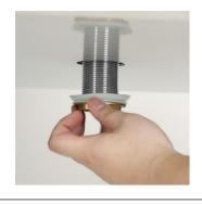
3. Turn the sink over, install over the drain hole. Wipe off the excess silicone at the bottom of the sink.
