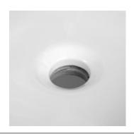
6. Wipe off the excess silicone around the drain. Allow silicone to dry 24 hours.
