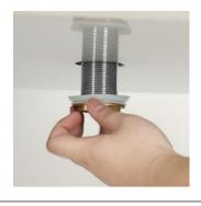
3. Turn the sink over, install over the drain hole. Wipe off the excess silicone at the bottom of the sink.
