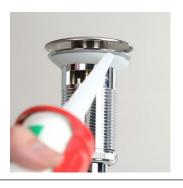
2. Apply the silicone around the drain hole at the bottom of the sink.
