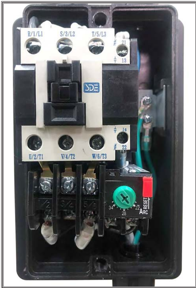
Figure 67. W1865 magnetic switch with cover removed.
