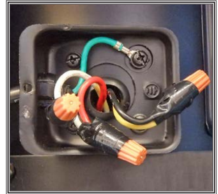
Figure 34. Motor wiring 240V.
