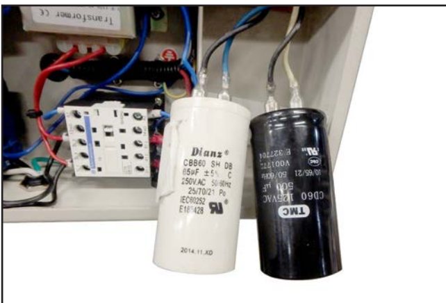
Figure 53. Start and run capacitors.
