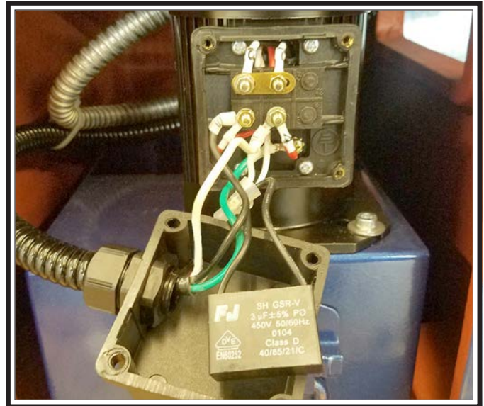
Figure 16. Coolant pump motor junction box.
