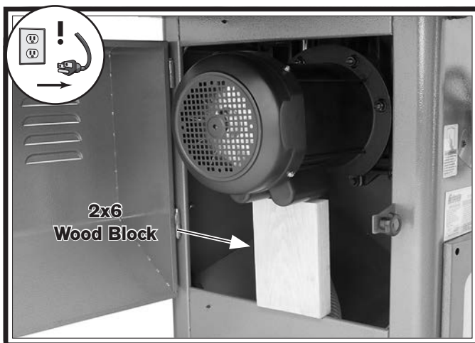
Figure 147. Motor resting on wood block.
