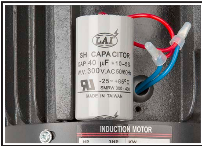
Figure 91. SB1101 run capacitor.
