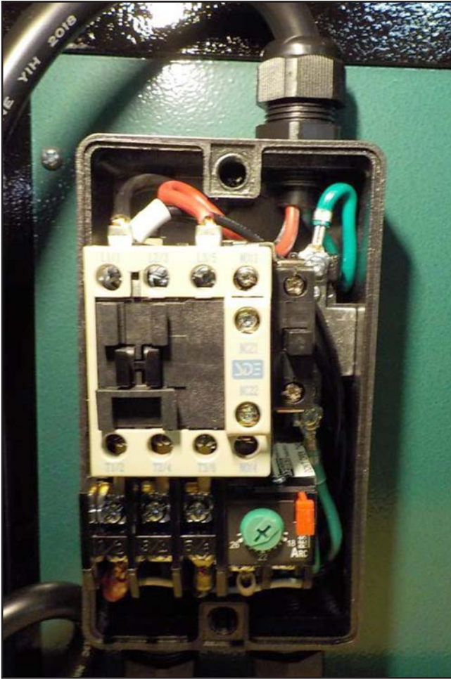
Figure 53. G1066R magnetic switch connections.
