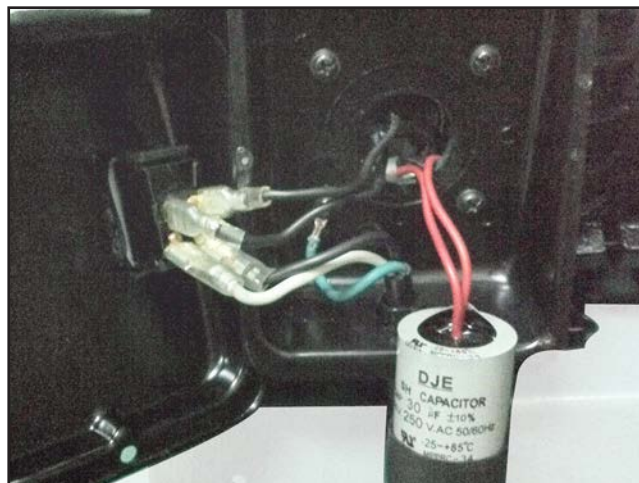
Figure 71. G0548ZP/G1029Z2P junction box, switch, and run capacitor.
