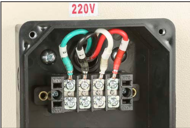
Figure 169. Incoming power wiring connections.
