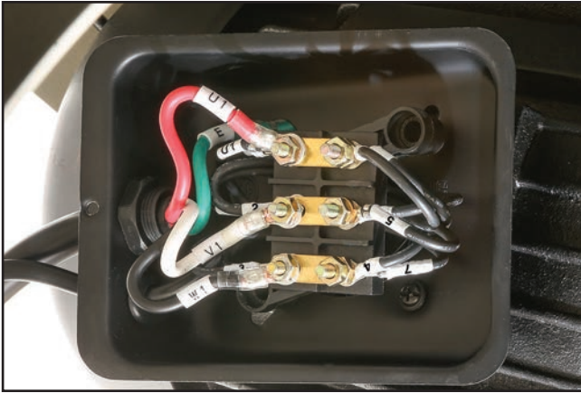
Figure 168. Motor wiring (220V).
