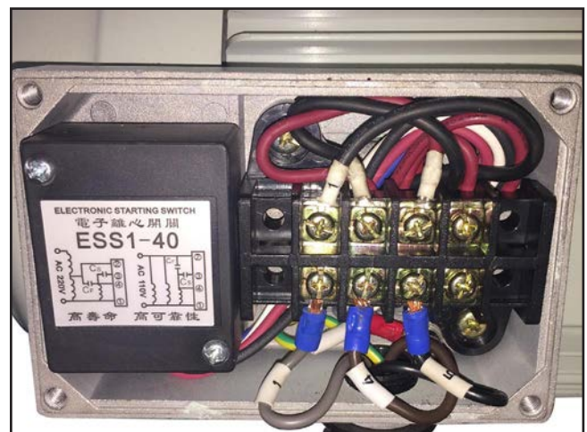
Figure 33. Motor junction box and starting switch.
