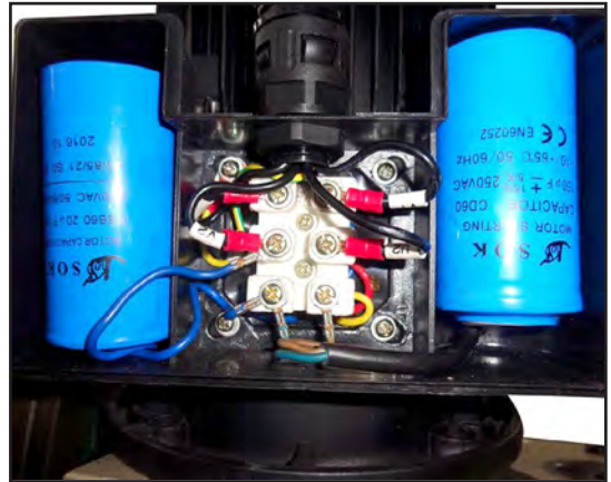
Figure 51. Motor wiring.
