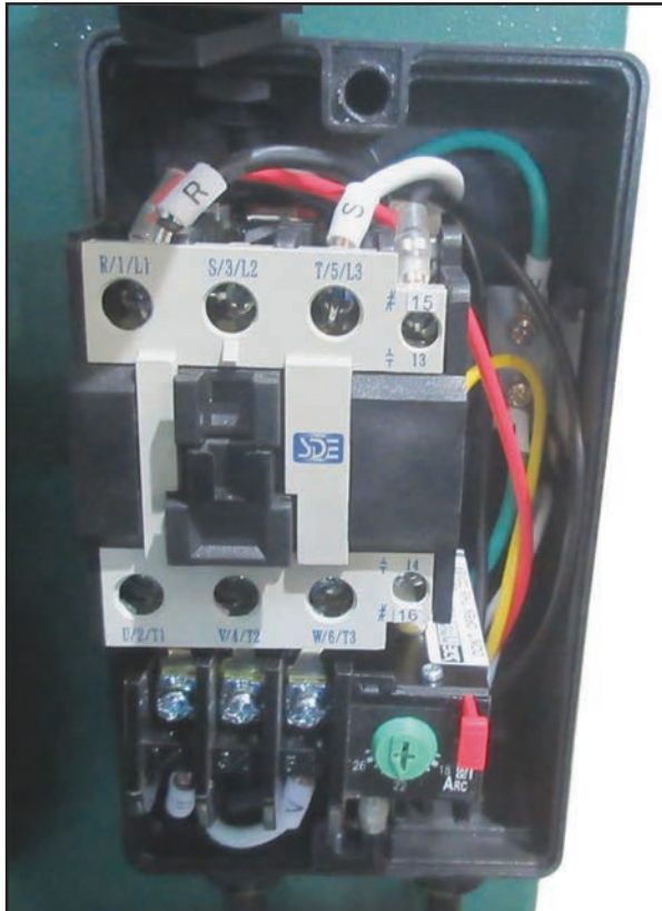
Figure 86. Magnetic switch wiring.
