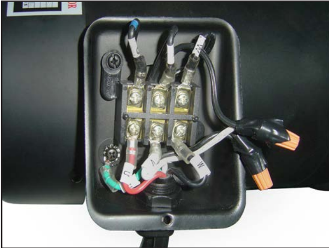
Figure 66. Motor wiring.
