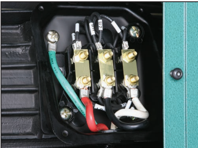
Figure 52. Cutterhead/feed motor junction box.
