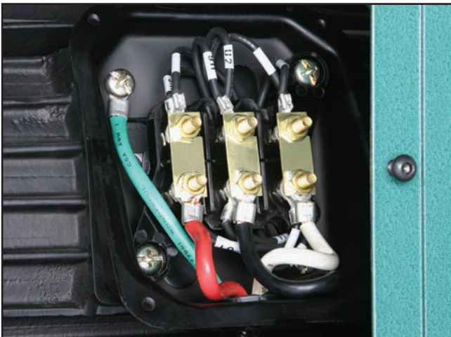
Figure 52. Cutterhead/feed motor junction box.
