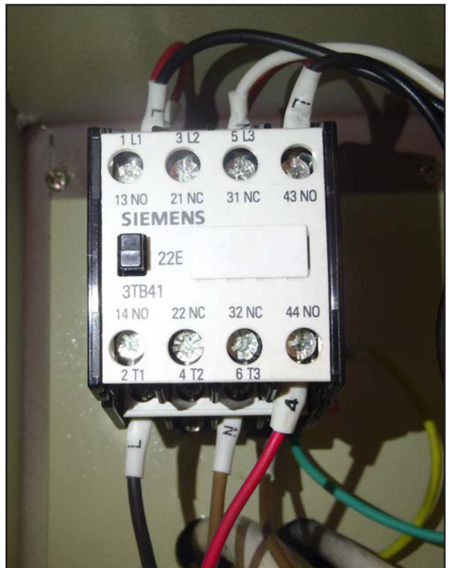
Figure 108. Magnetic contactor.
