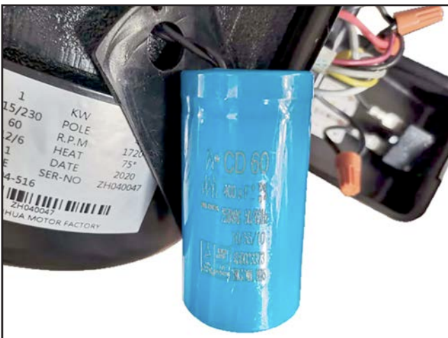
Figure 76. Capacitor wiring.
