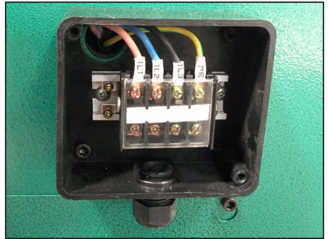
Figure 80. Power-in junction box connections.
