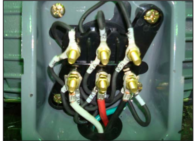
Figure 92. G0450 480V sanding drum motor wiring.
