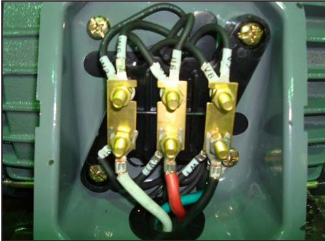
Figure 91. G0450 240V sanding drum motor wiring.
