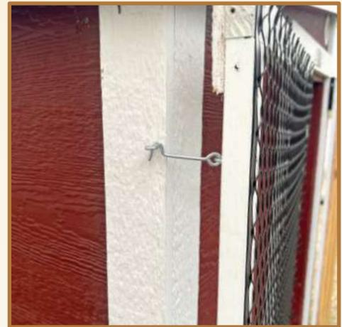
**3.** Attach eye hook to the right side of the man door trim using the same method as step #2.
