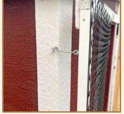
**3.** Attach eye hook to the right side of the man door trim using the same method as step #2.
