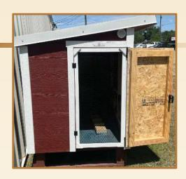
2. Attach the eye hook to the corner trim. With the screen door open use the hook latch to mark the location for the eye hook. Pre-drill hole with 1/8-inch drill bit. Screw the eye hook into the pre-drilled hole.
