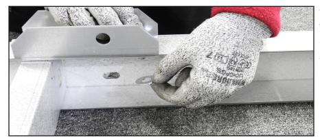
Where there is no cross-channel at the fastening location of the mounting bracket use a 3/8 washer as a spacer.
