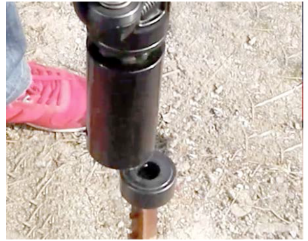
Fig. 4 ) Insert Inner Post Head \Phi 67 . Use a wood handle or metal bar to force inside Sleeve.
