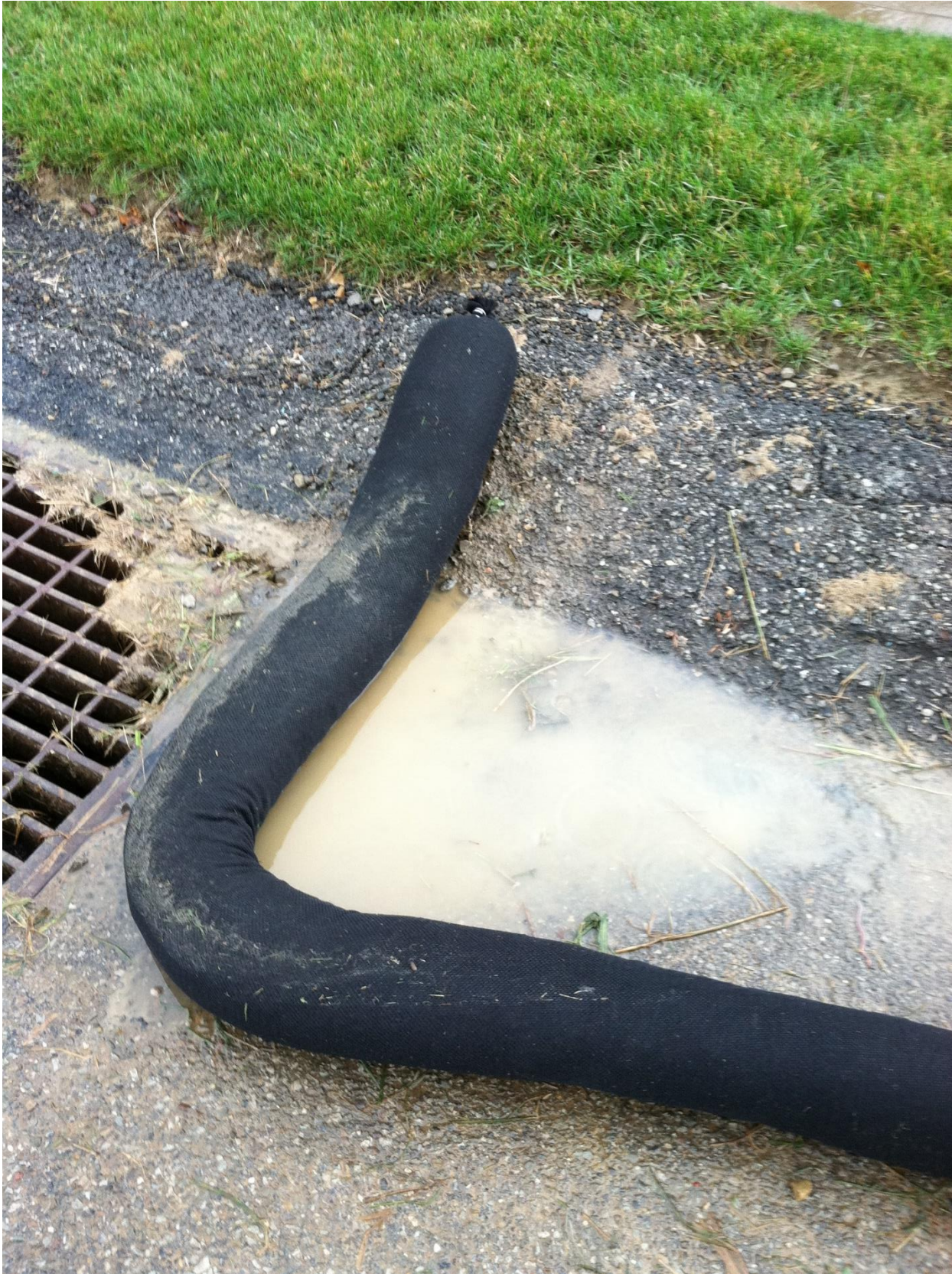
Pictures from R&D field testing
