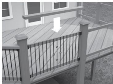
**5.** Attach cap rail as desired for finished appearance.
