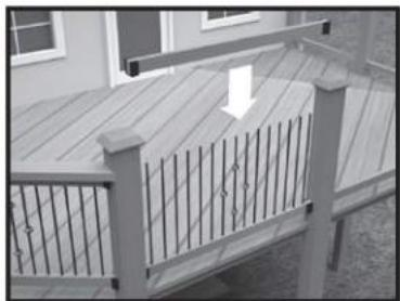
6. Once all balusters are set over bottom rail Mega EZ Mounts or into Mega Shoes, set the top rail by appropriately aligning the balusters with the top rail Mega EZ Mounts or Mega Shoes. Attach top rail to support posts on each end using Fortress Rail Bracket (sold separately).
