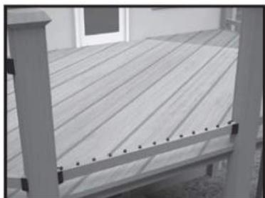
4. Attach bottom rail to support posts on each end using Fortress Rail Bracket (sold separately).
