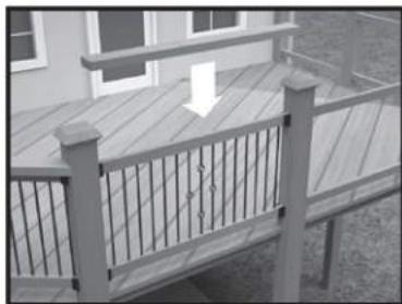
7. Attach cap rail as desired for finished appearance.
