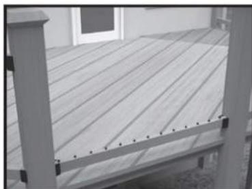
4. Attach bottom rail to support posts on each end using Fortress Nylon Rail Bracket (sold separately).
