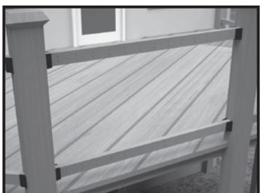
**3.** Attach bottom rail and top rail to support posts on each end using Fortress Rail Bracket (sold separately).
