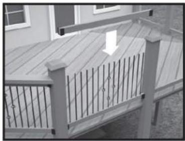
6. Once all balusters are set over bottom rail EZ Mounts or into RP Shoes, set the top rail by appropriately aligning the balusters and top rail EZ Mounts or RP Shoes. Attach top rail to support posts on each end using Fortress Rail Bracket (sold separately).
