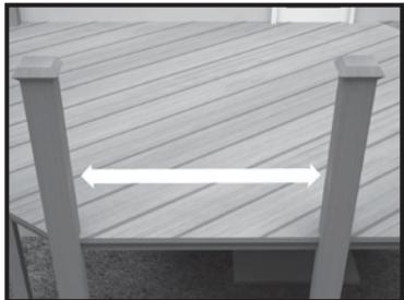
**1.** Measure the opening from post to post to determine length of baluster rail section. Cut top and bottom 2x4 rails to appropriate length.
