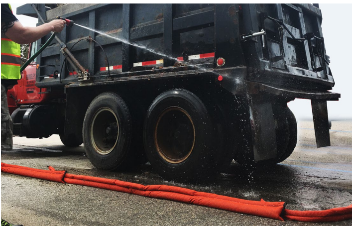
Truck Washout—set up quick wash off sites to contain water
