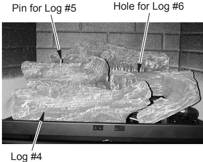
Figure 18 - Installing Log #4
