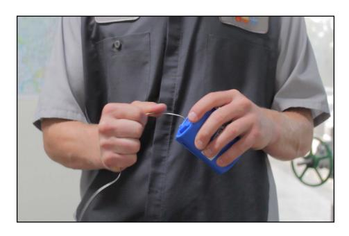
3. SECURE THE FREEZEPRO® FROST PROTECTION JACKET BY LACING THE SS WIRE BACK AND FORTH BETWEEN THE SS LACING HOOKS:
