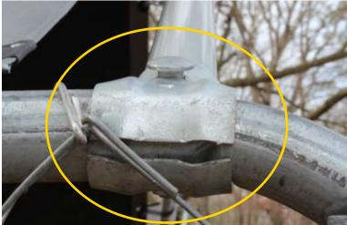
**7)** Place framework over the kennel and attach each of the 4 roof pipes using the single sided clamps. Please note that the frame measures less than 10 ft in width and length to attach to the point on the kennel before the curved corner sections.
