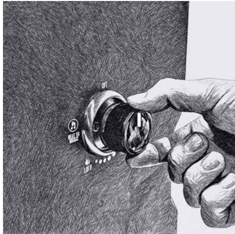
[Figure 3] - Turn gas control to "OFF".
