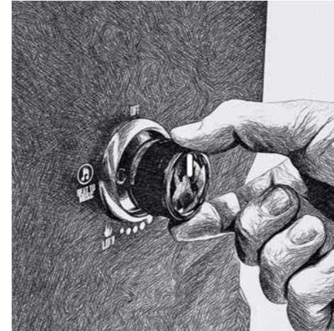
[Figure 6] - Turn gas control to "OFF".
