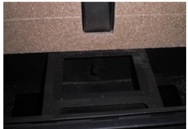
Figure 32: Burn Pot Cradle/Igniter Tube
