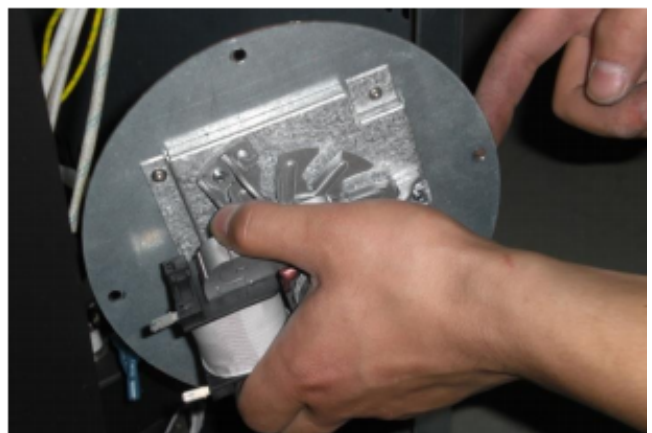
Figure 34: Combustion Motor Assembly
