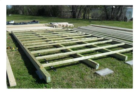
2) Kits include small treated floor joists. The technical details will indicate to lay then flat or stand on end. Laying them flat or on end will change the distance to the outside edge. The walls will overhang the treated joists by approximately 1/8" if done correctly
