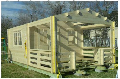
6) Install storm straps to outside corners behind the horn. Place the single hole at the top log and secure and tighten the bolt. In the two lower slotted holes, install bolt AT THE BOTTOM OF THE SLOT and finger tighten only. Now remove ratchet straps and the logs will not open, but allow shrinkage.
