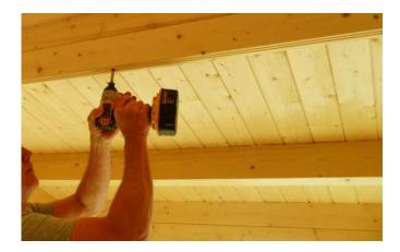
8) Exterior & Interior trim boards are not fastened to wall logs. (NO NOT NAIL OR SCREW TRIMS TO WALL LOGS) They trims create a trough only for the wall logs to move
