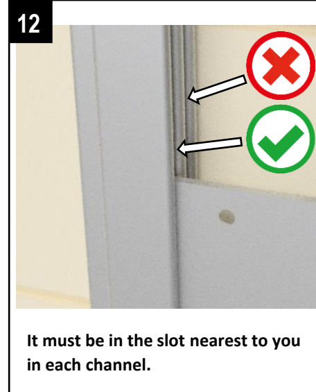
Slide the door panel with grommet down the channels.
