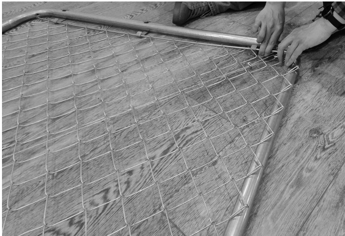
(#1) The remaining mesh section to install the tension rod to (#2) The excess mesh to be discarded
