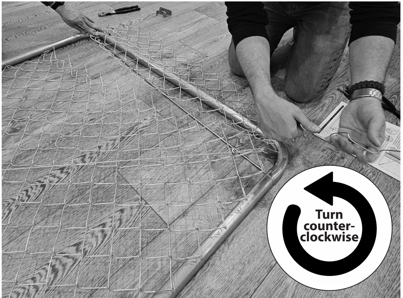
At the top of the frame: Cut right before the knuckle loop
